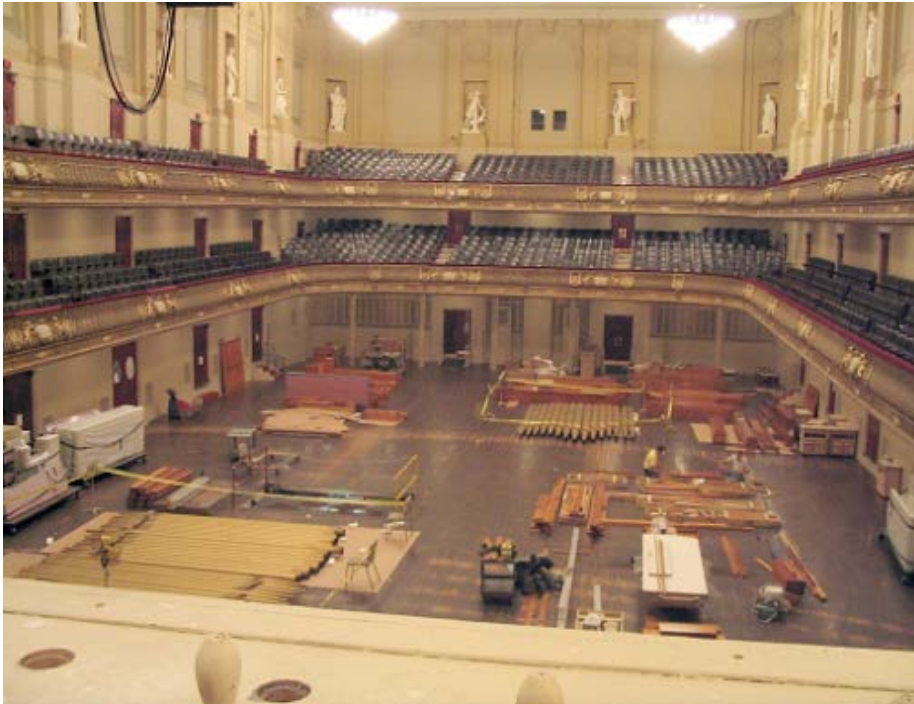
Organ pipes on concert hall floor, awaiting re-installation. Photo taken from bare organ chamber above the stage.
